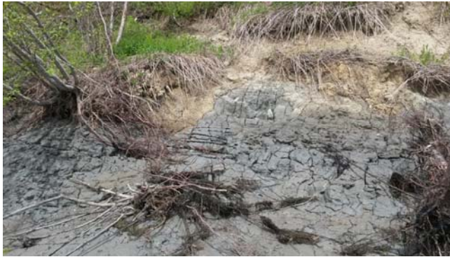
Figure 5-2 Photograph of Existing Slope
